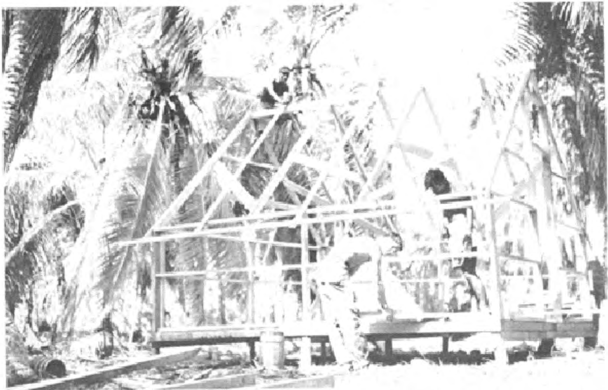
Figure 3. Navy Construction Battalion personnel, assisted by Marshallese, construct wooden house frames on Rongerik for Bikinians.
