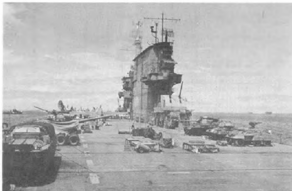
Figure 14. Armored vehicles and other Army equipment aboard USS Saratoga (CV-3), ready for exposure to atom bomb, CROSSROADS.
